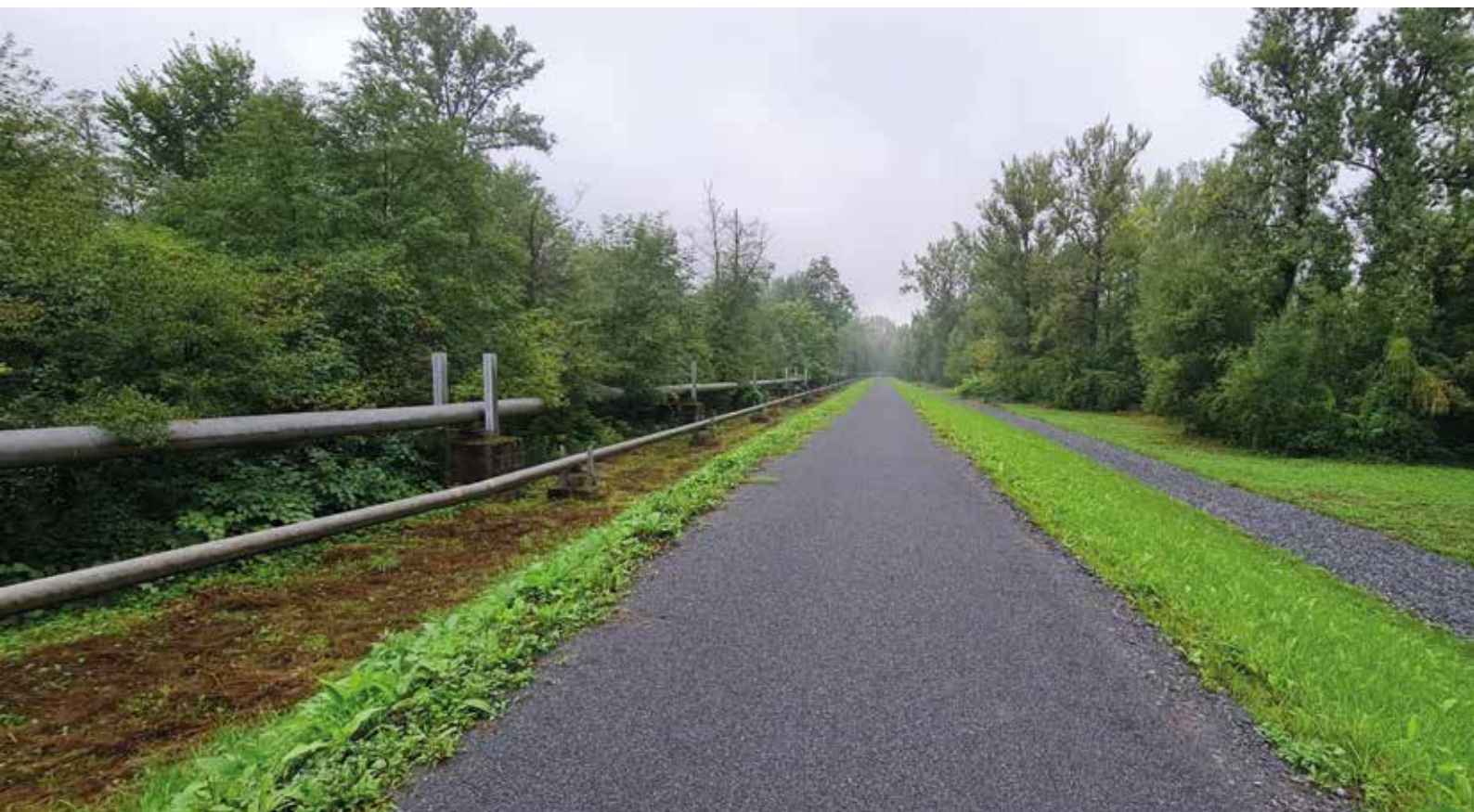
LB dyke along the Ostravice River in Paskov after construction
