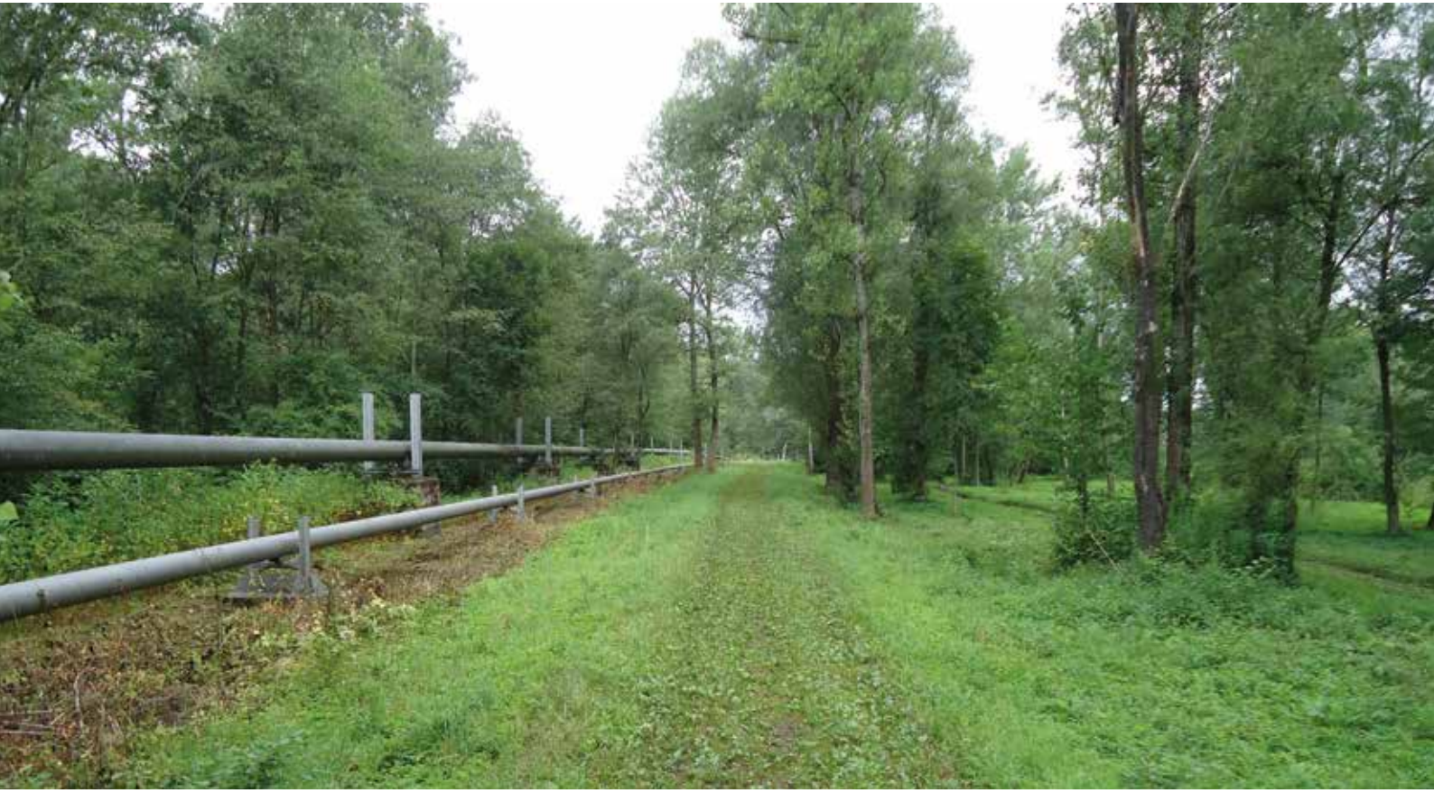
LB dyke along the Ostravice River in Paskov before construction
