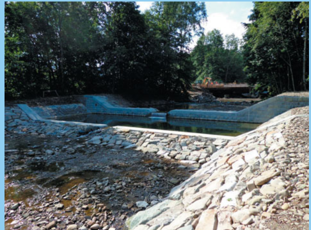
Mohelnice – The general view of the Object 1 after the finalisation
