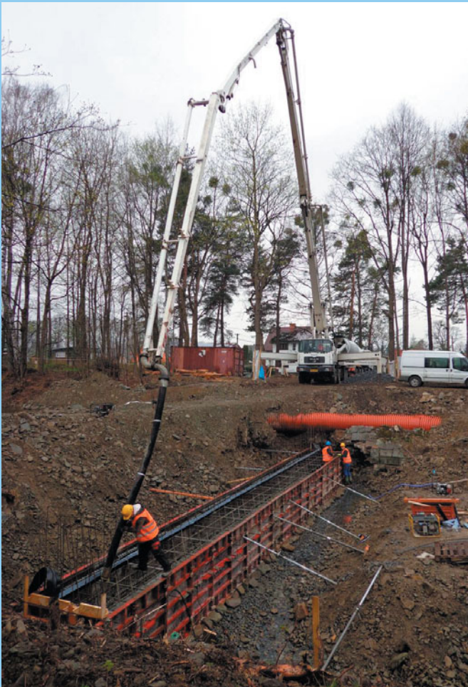
Mohelnice – The concreting works
