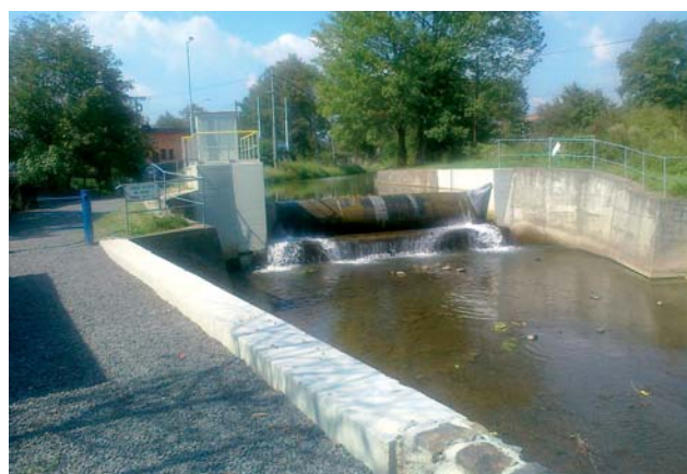
Porubka Creek – The new ogge weir
