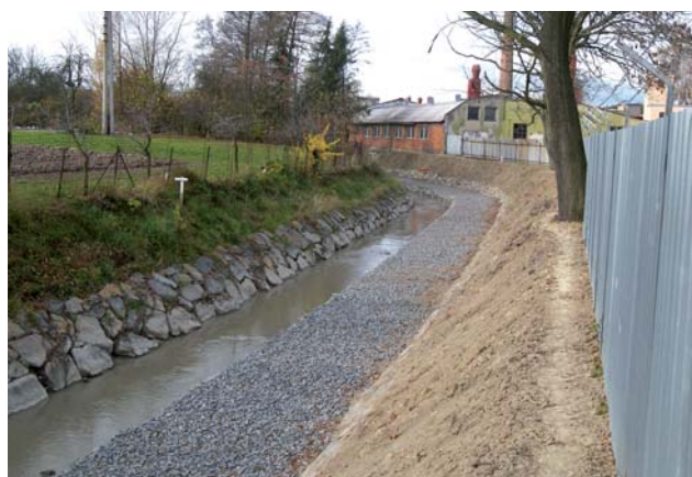
Porubka Creek – The finished section of the strengthened berm
