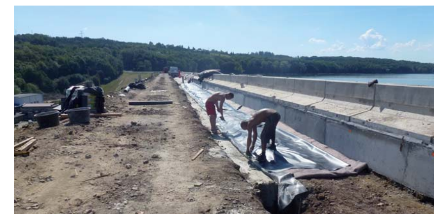
Reservoir Těrlicko – Laying of hydro-insulating sheets
