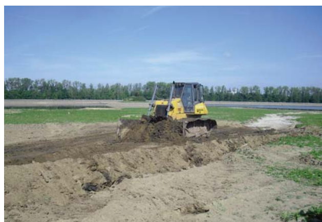
Reservoir Baška – Excavation of sediments
