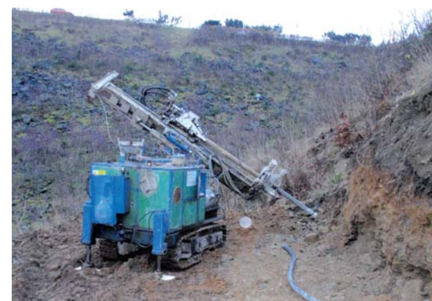
Reservoir Šance – Draining gallery / slope nailing above the construction pit
