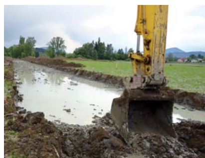
Reservoir Baška – Excavation of the draining river bed
