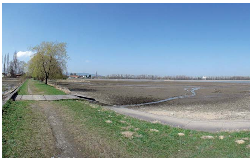
Reservoir Baška – General view over the area for the excavation of sediments before the start of the event
