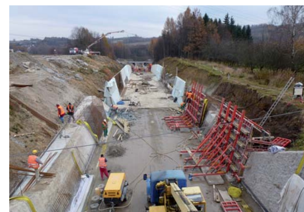
Reservoir Těrlicko – Construction of a new chute
