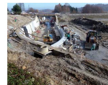
Reservoir Těrlicko – The overflow repairs
