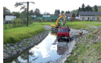
Porubka Creek – Slope adjustments
