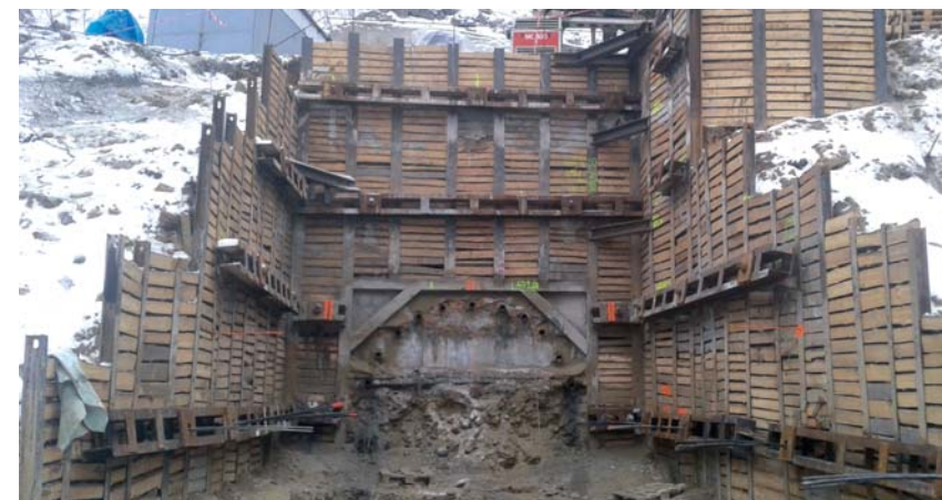
Reservoir Šance – Draining gallery / the construction pit – the micro stillt cover
