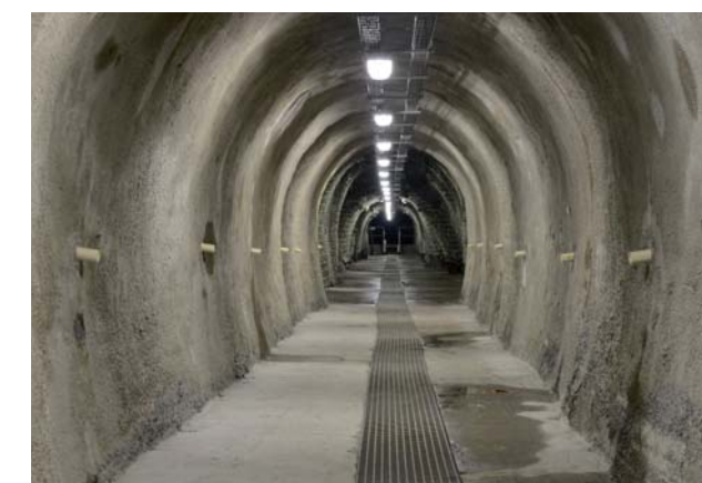
Reservoir Šance – Draining gallery
