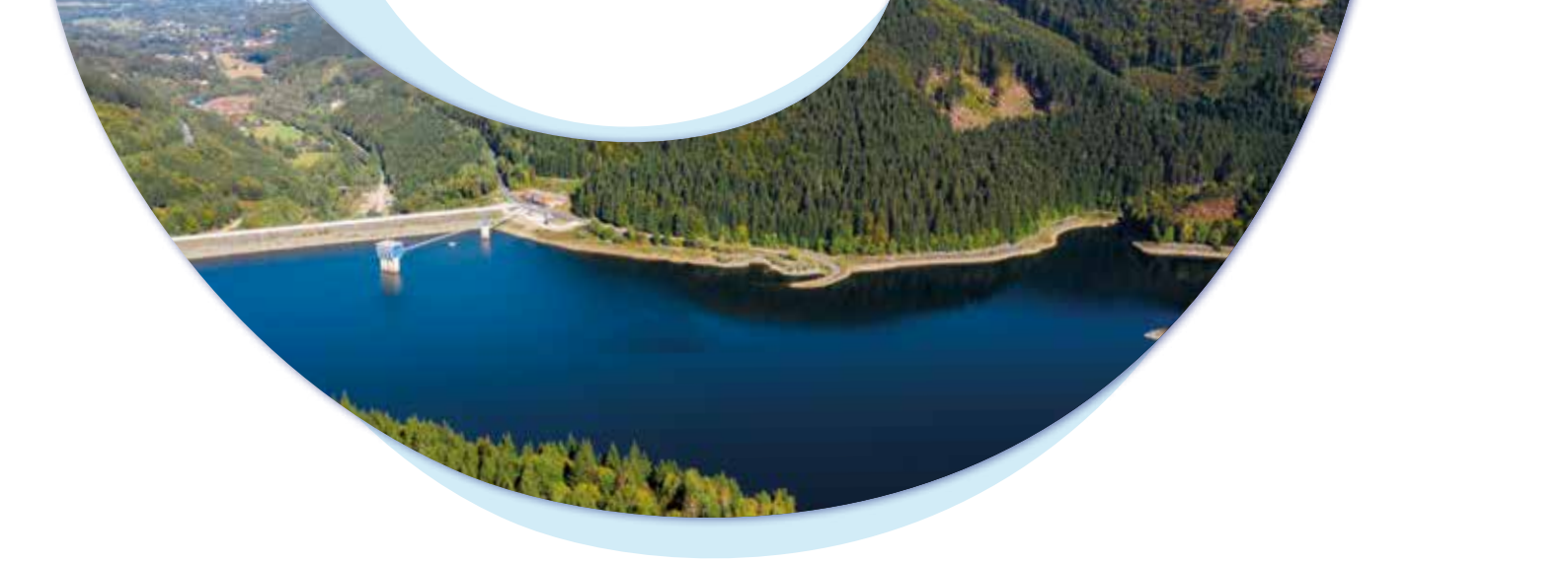
Photo: Waterworks Šance after reconstruction
